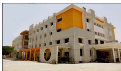
Poornima College of Engineering (PCE)
